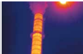
Refractory material inspection on a furnace chimney.
