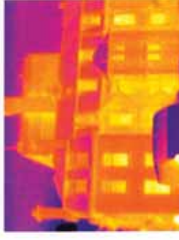
Building Services Find hot spots due to poor insulation
